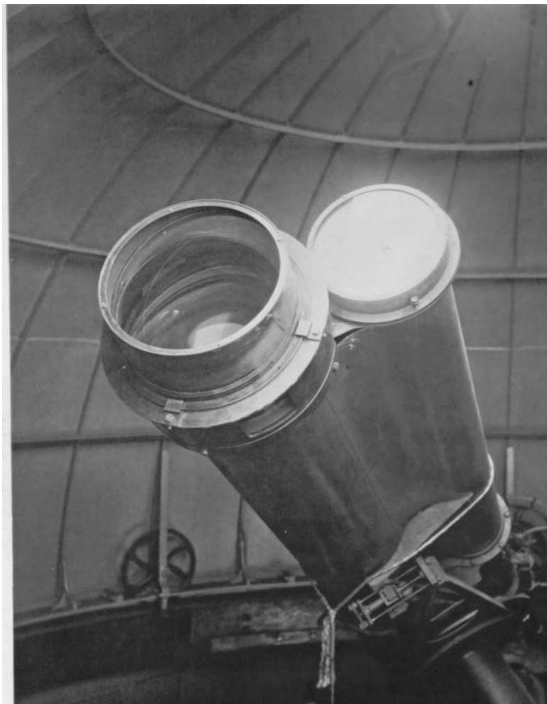
Figure 5.3. Francis McLean's objective prism mounted on the Cape Observatory astrograph, 1898. The prism aperture is 12 inches.
