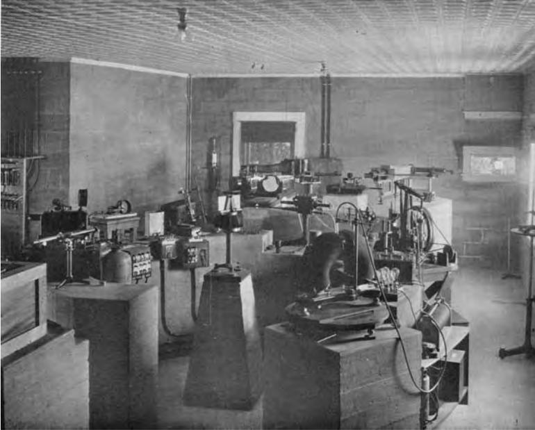
Figure 4.17. The Snow telescope spectroscopic laboratory at the Mt Wilson Solar Observatory, 1906. A quartz spectrograph is just above the concave mirror. To the right of this is a Hilger one-prism spectrograph. The main instrument is the Littrow spectrograph with a plane Michelson grating,  $8.3 \times 4.4$  cm, with 7000 gr/cm.
